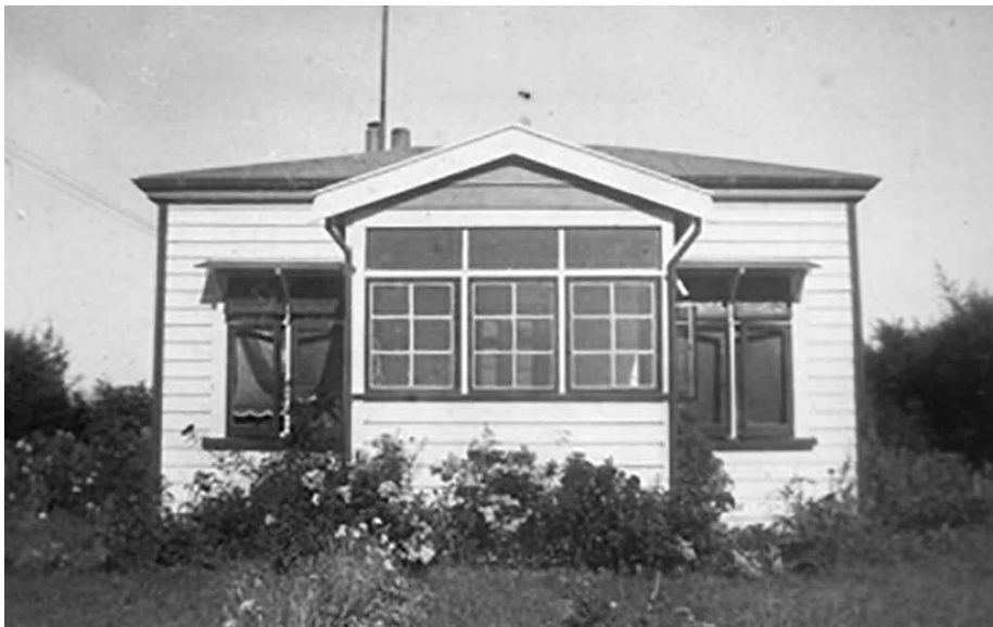
The Battersea cottage. Paul and Hilda's first home was purchased for £75 in 1920 and shifted from its original site in Greytown to their farm at Battersea, a distance of c. 6 km. Transportation was via a flatbed with the house on it drawn by a traction engine and winch. The traction engine would proceed ahead and then winch the house up to it, and repeat the process many times on the way to its destination.
